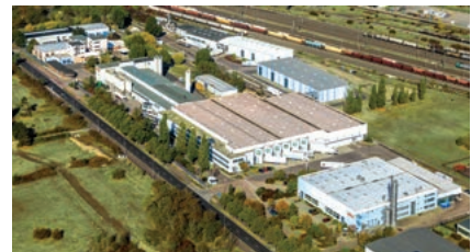
Plant in Lutherstadt Wittenberg
